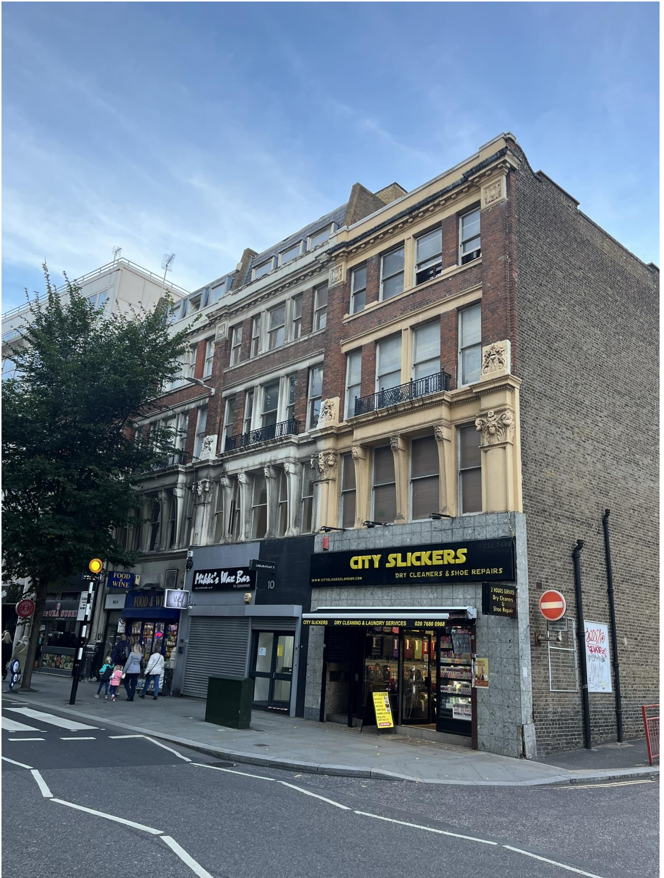
The four adjoining Victorian buildings at Nos. 6-12 Minories are attractive contributors to the architectural character of the area, but remain unlisted (Credit: SAVE Britain's Heritage)
