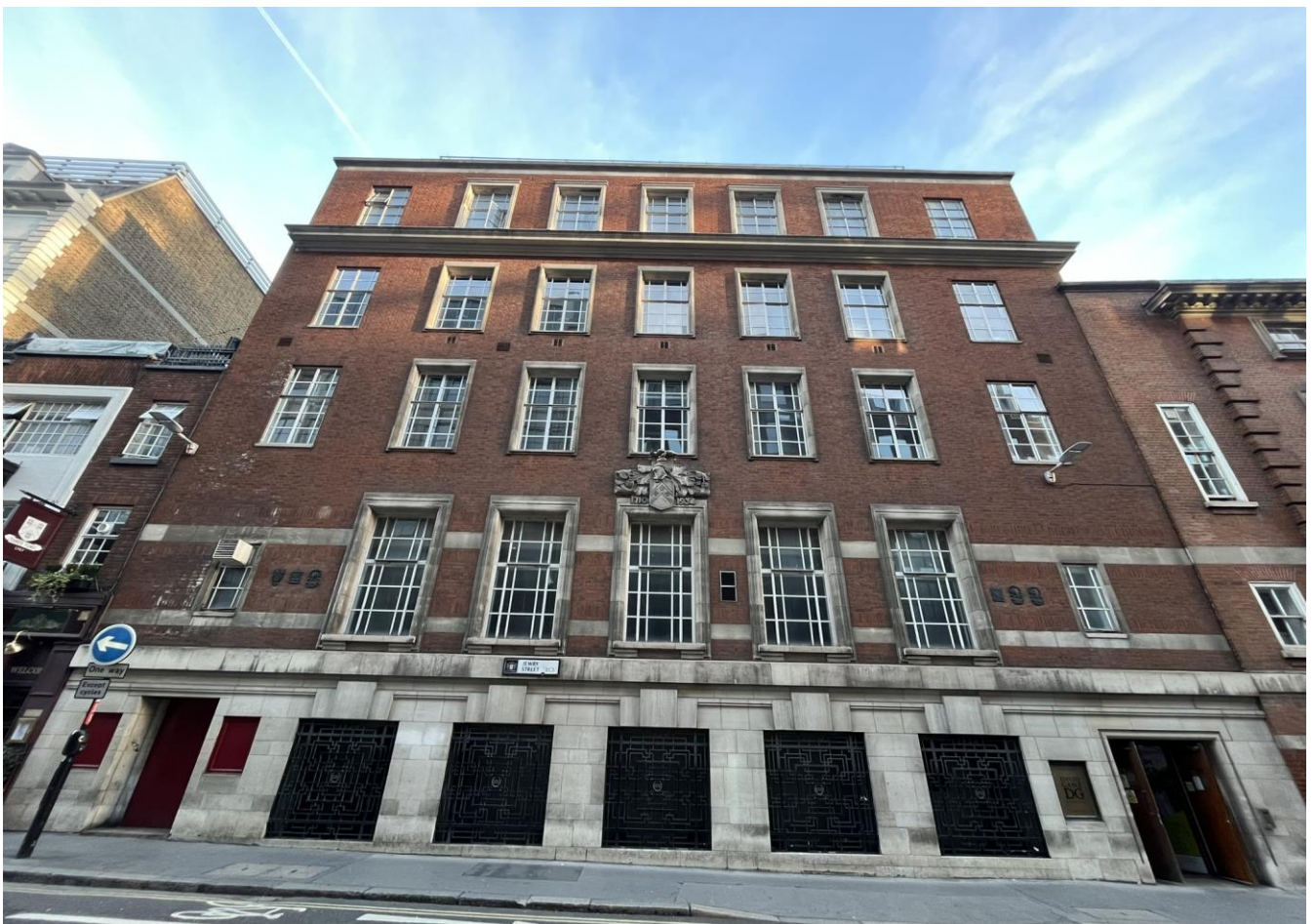
The northerly extension added to the Sir John Cass Institute in 1954 is an attractive landmark designed by Verner Rees (Credit: SAVE Britain's Heritage)
