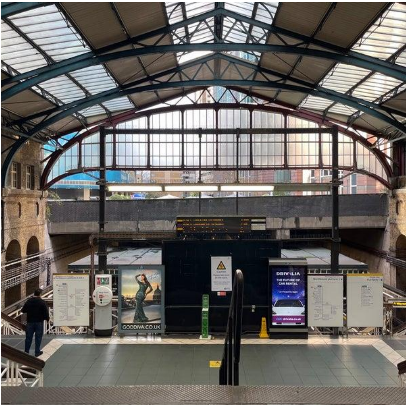
View looking north within the Victorian trainshed of Aldgate Underground Station, completed in 1876, with the cast iron span roof over the four platforms below (Credit: SAVE Britain's Heritage)
